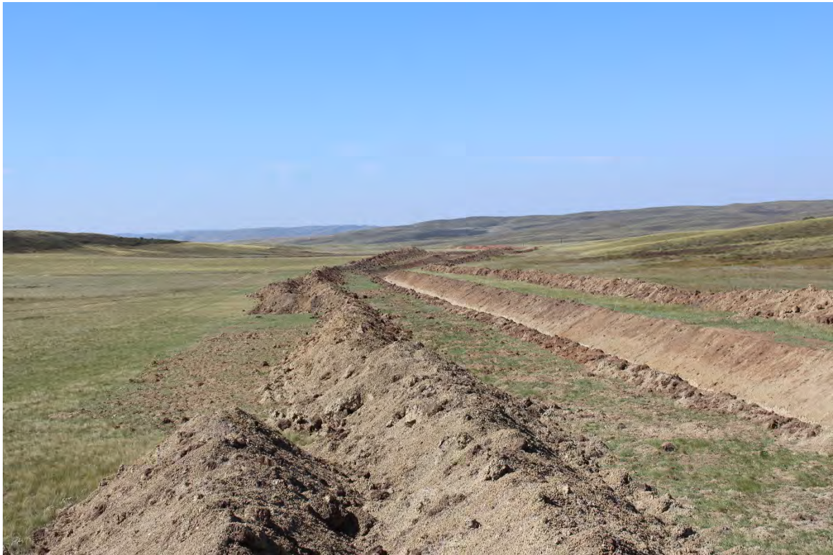
Figure 4.14: Waste Dump Diversion Channel (Photo 7)
